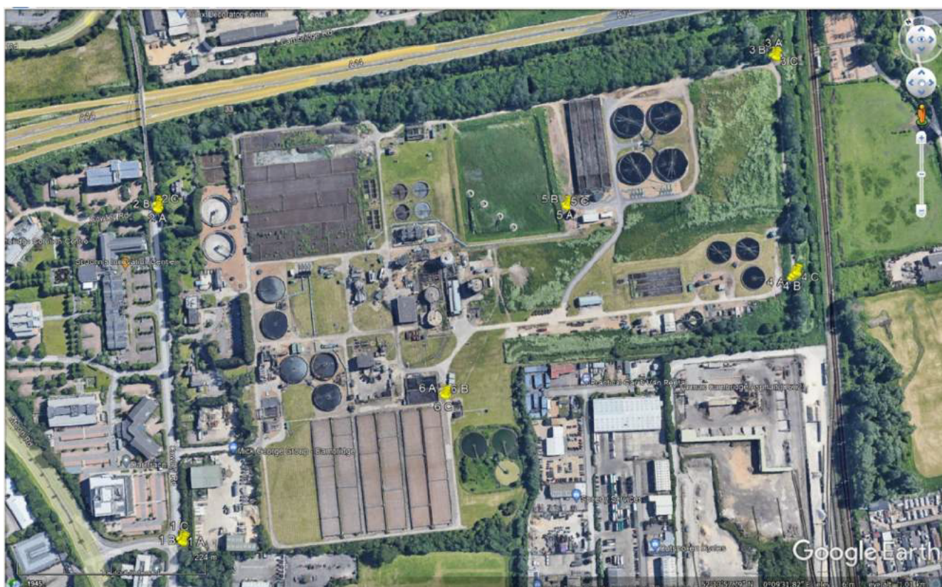
Figure 8: Aerial image of Cambridge WWTW Relocation Project pinned survey area within current boundary (image from Google Earth)
